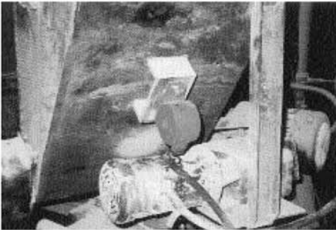
SILENT Turbine mounted to a fly ash chute to keep ash flowing.
